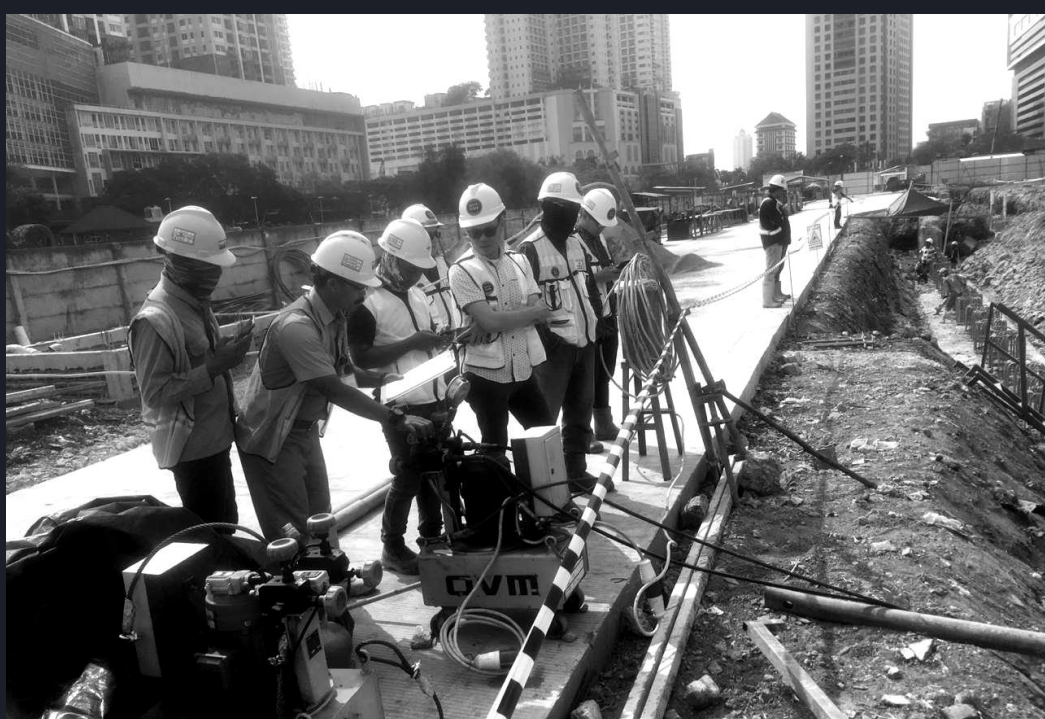
JOINT INSPECTION PROVING TEST GROUND ANCHOR
