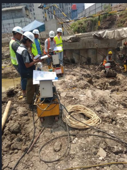
JOINT INSPECTION: CHECKING THE GROUND ANCHOR
